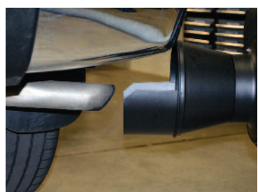
The high-output suction fan captures fumes and safely discharges them up to 30’ away, using the hose provided.
